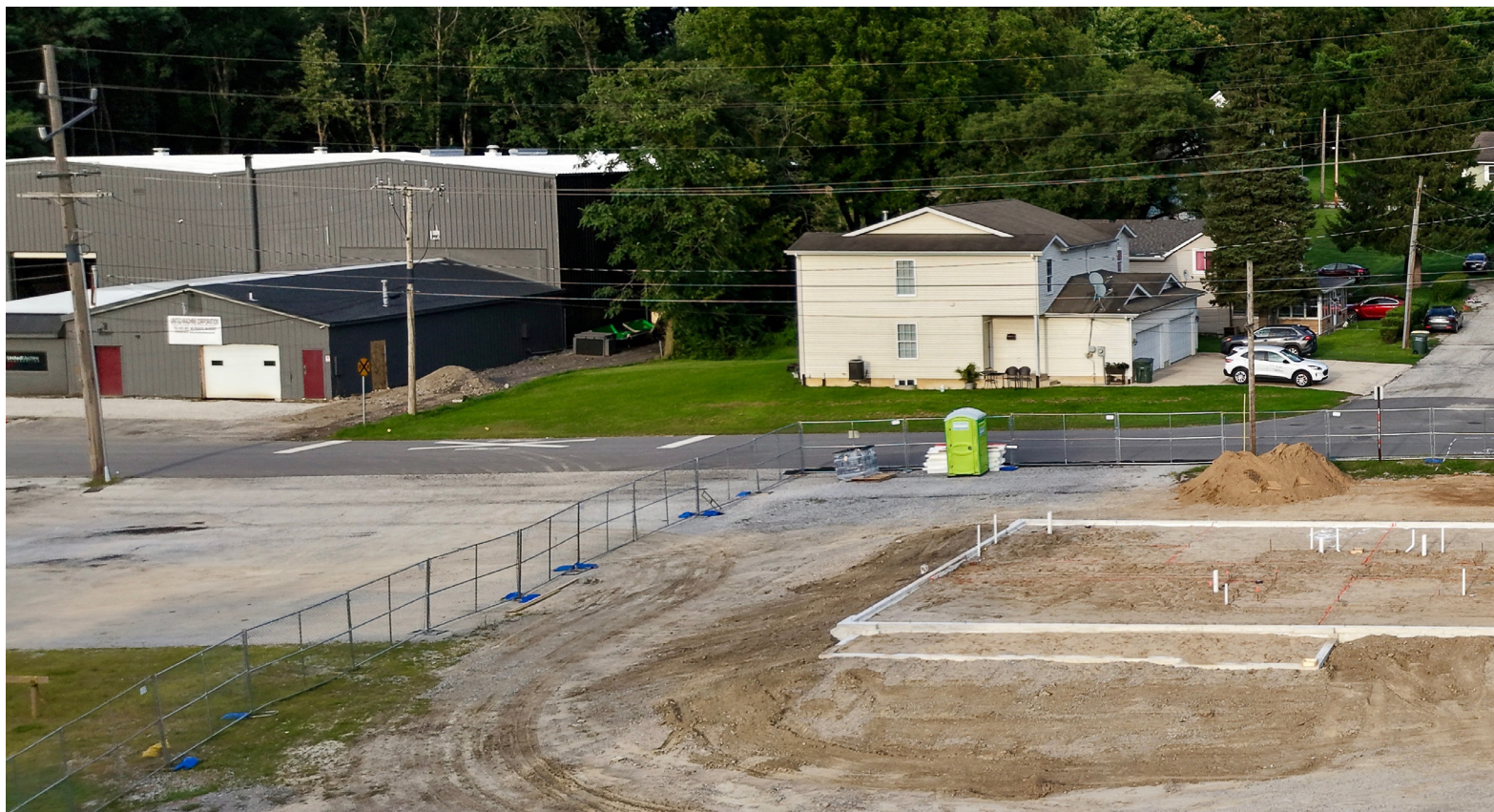
Following rough-in plumbing, we prepared The Crossing for flatwork.
