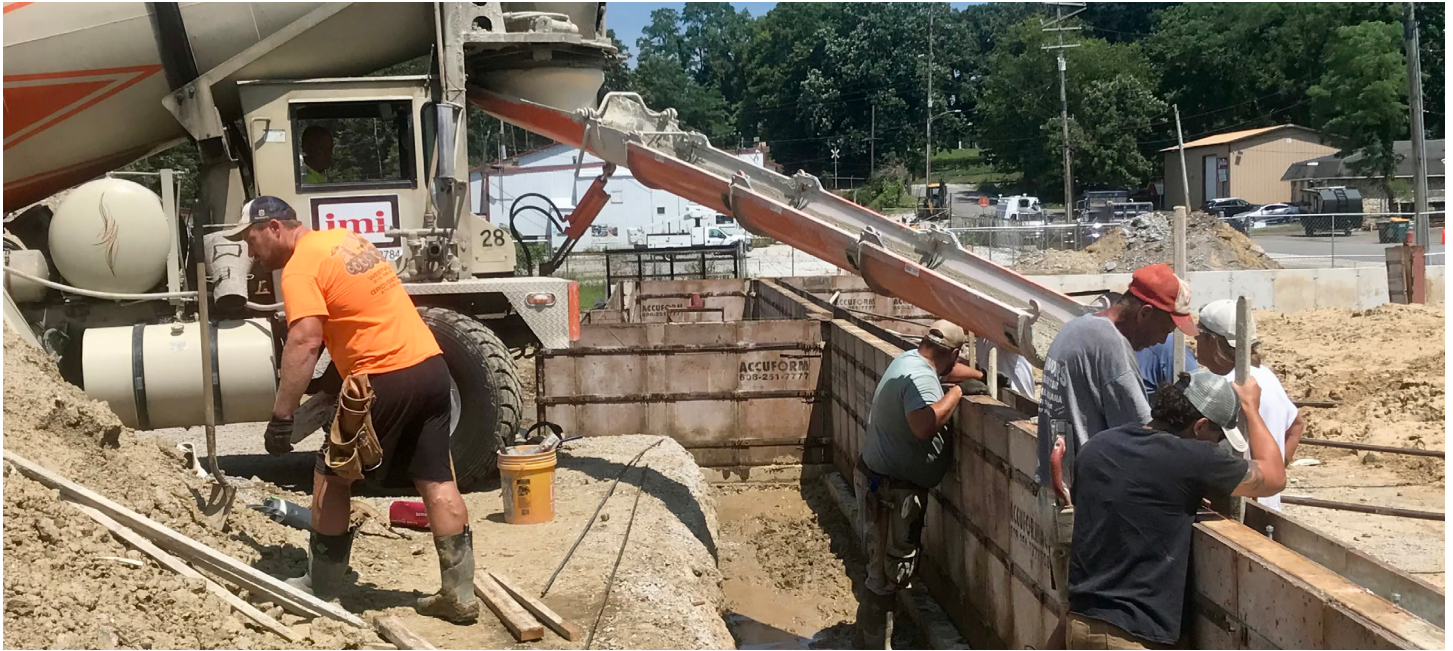
Pouring the foundation at The Crossing.
